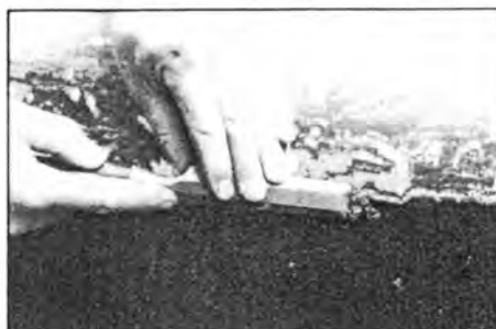
The paint is so thick here that chiselling was the best way. Keep the blade as flat as possible to minimise the risk of digging through to the gel coat.
