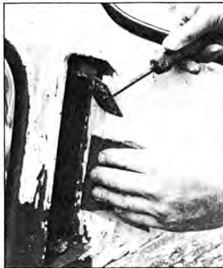
Using paper or a multi-sided scraper for the awkward bits.
