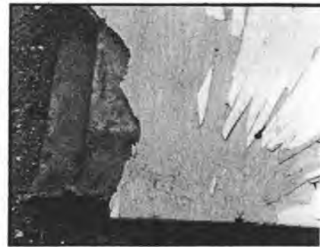
Part of an Elan boot lid after an accident showing extensive gel cracks and paint peeling off between the gel crack lines.
