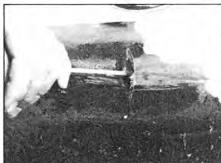
Scrape the paint off using a multi-sided scraper.
